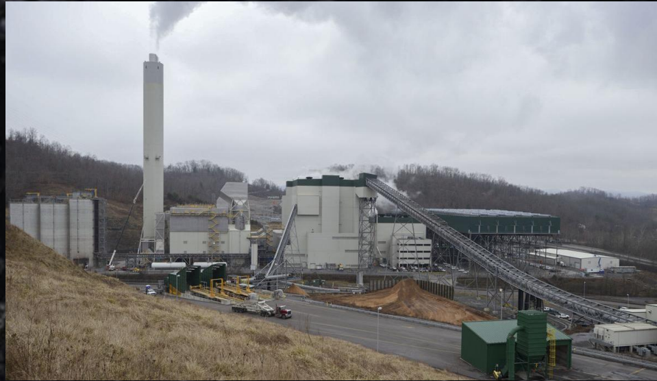
Virginia City Hybrid Energy Center burns coal, biomass, gob-pile coal
